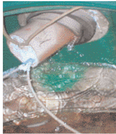
Degraded entry boots and leaking entry seals are common problems found by operators.
