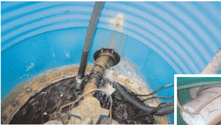
Degraded entry boots and leaking entry seals are common problems found by operators.
